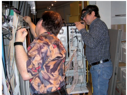
Figure 4.30. Setting up one of the first VLBI Standard Interface (VSI) based acquisition systems for unformatted VLBA sampler at 1 Gbps.
